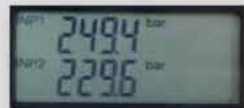
Screen shot showing two inputs. Pressure 1 and 2.
