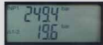
Screen shot showing differential pressure
